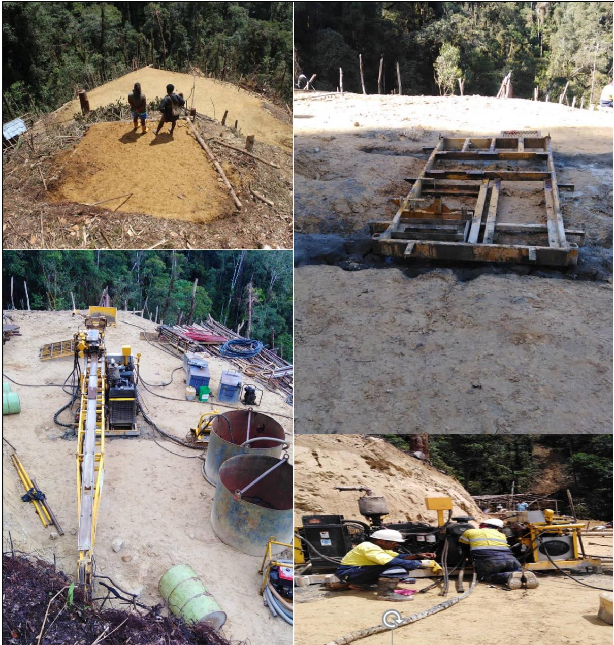
Figure 4. MCD008, drill site clearing and rig assembly
