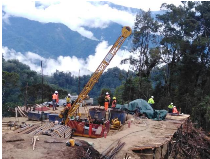
Figure 3. Drill Rig set up on MCD004
