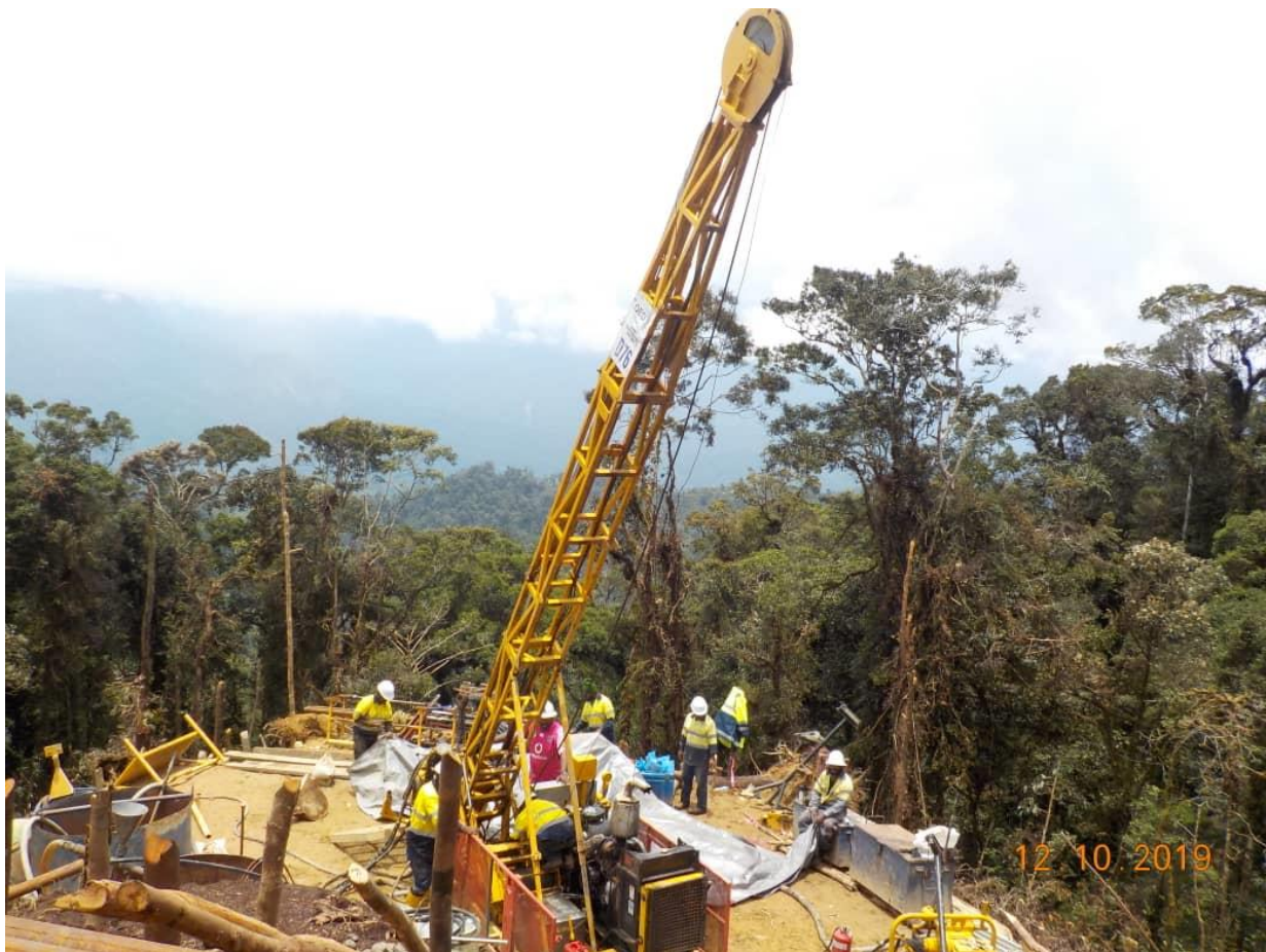
Figure 2: Drill rig set-up as of 12 October.
