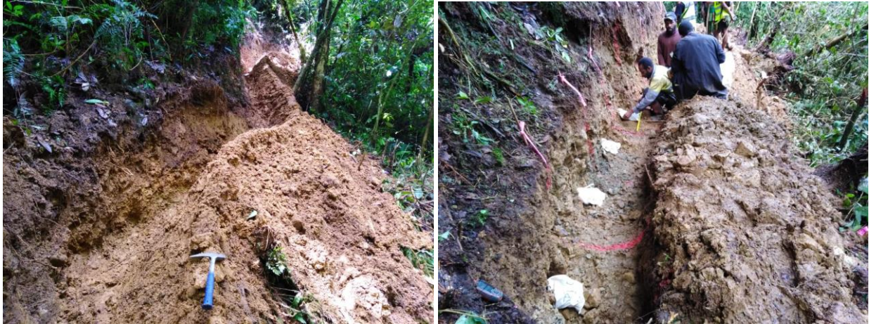
Figure 3: Trenching Activities currently underway at Mongae Creek
