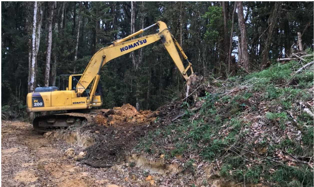
Figure 3: A Komatsu PC200, costeaming along the top of ridges and their flanks forming the headwaters to the drainage at Crown Ridge
