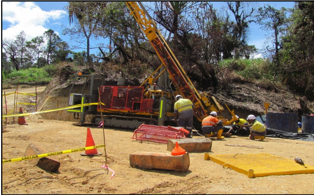
Figure 4: QED’s Atlas Copco CS14 Drill Rig on drill hole CRD001
