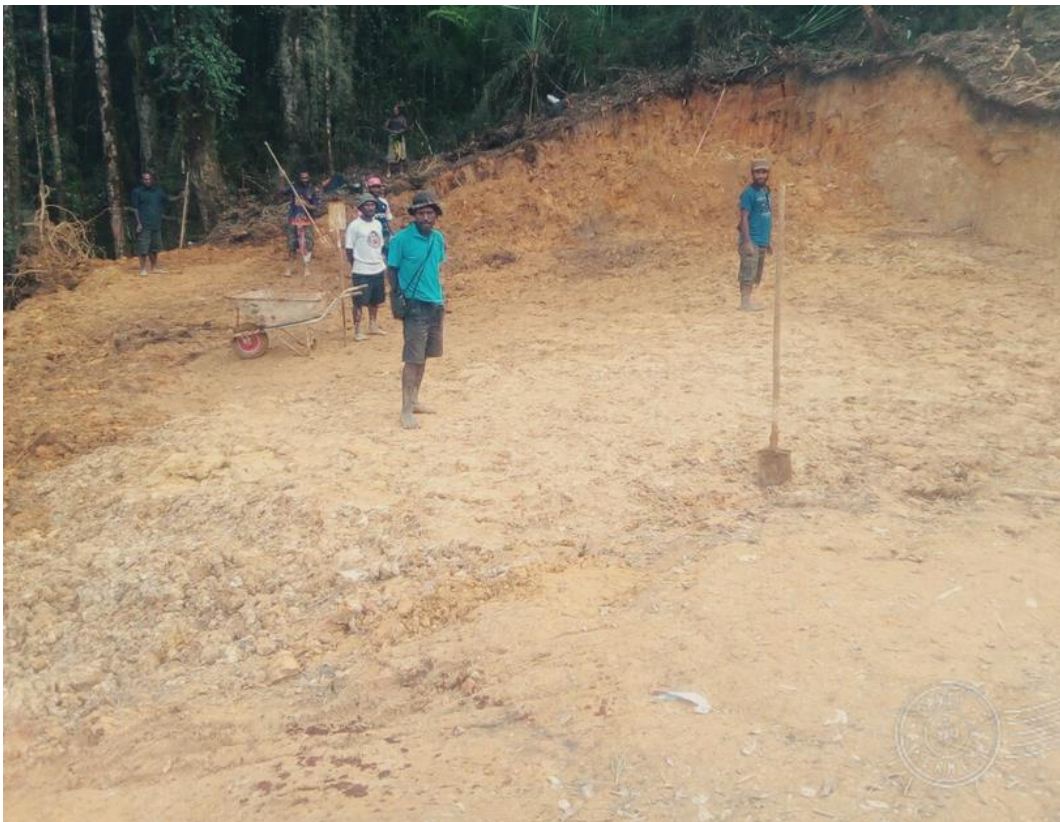
Figure 5: Prepared drill pad ready for rig mobilisation
