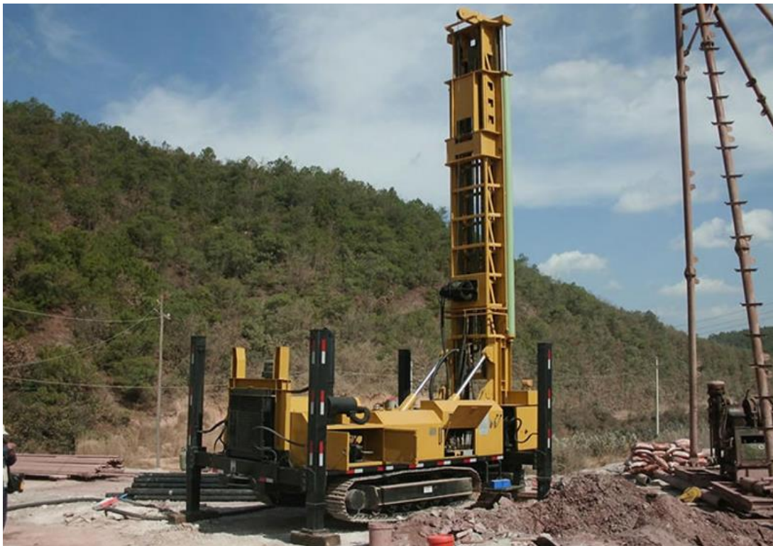
Figure 6: Equipment mobilisation (Atlas Copco CS14 Drill Rig)
