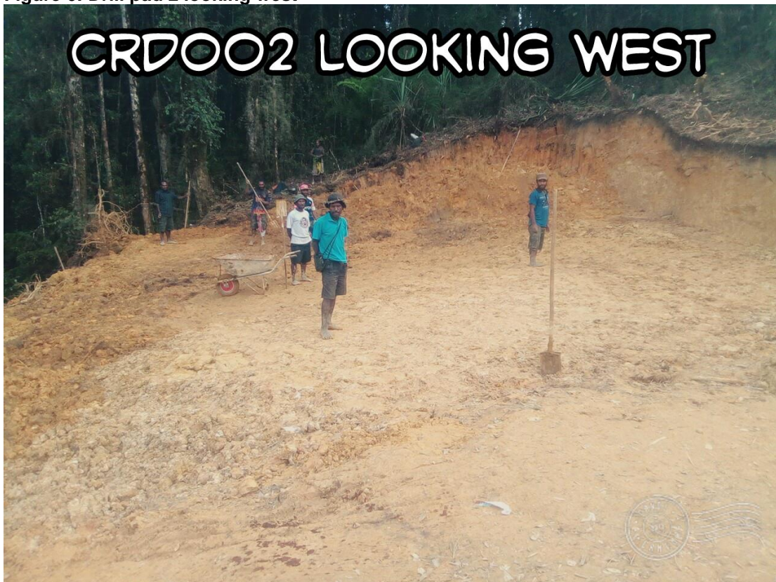
Figure 6: Drill pad 2 looking west
