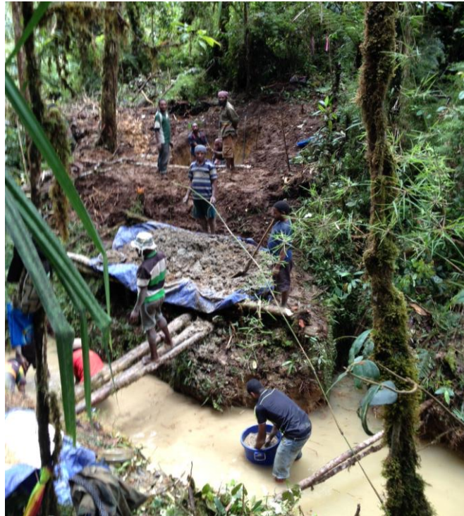
Figure 6: Ongoing works at Crown Ridge Gold Project
