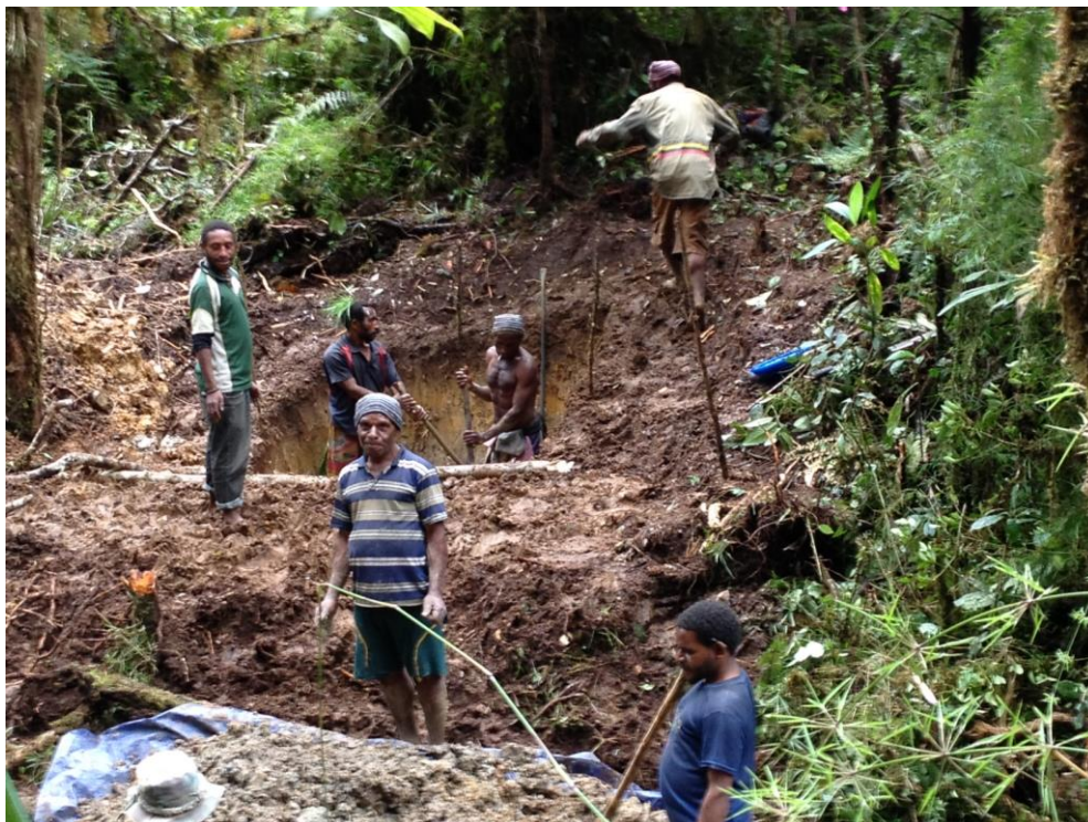
Figure 7: Ongoing works at Crown Ridge Gold Project
