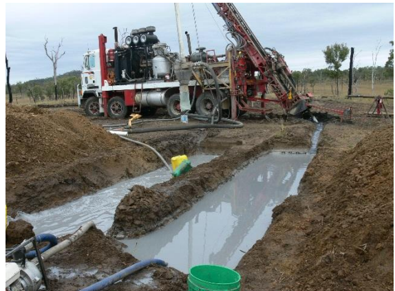
Prior Trenching at 'Black Bullock'
