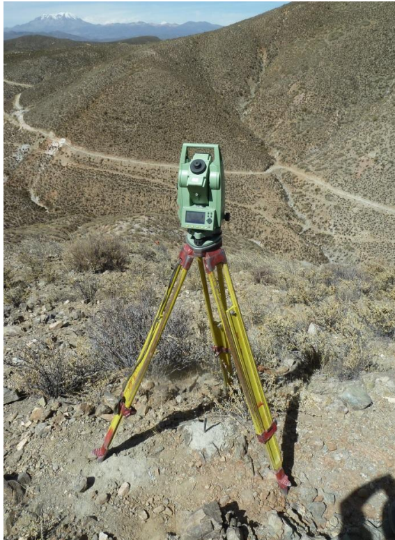
Goldsmith Resources SAC's upgrade to the road to Eladium Mine underway
