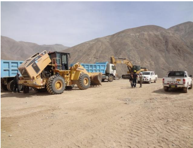
Stockpiling bulk sample ore for the April commissioning of the Peruvian gold plant.
