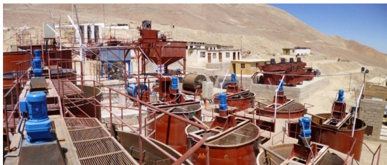
The Mollehuaca Gold Plant Peru: Production soon.
