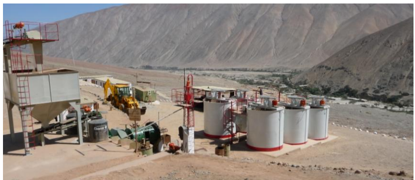
Existing Mollehuaca CIL plant
